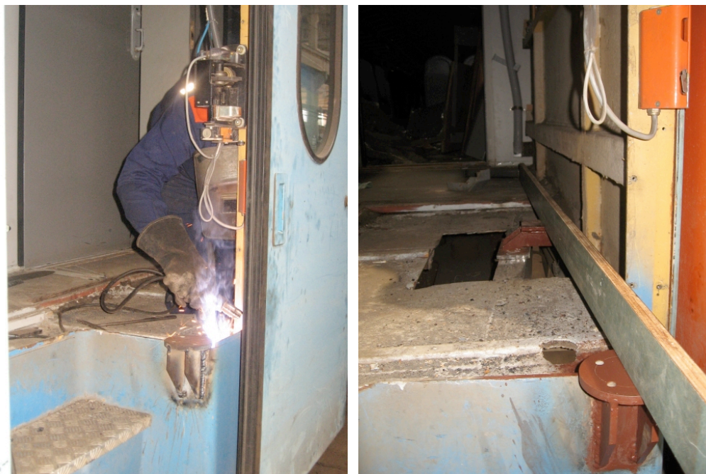
fig. 8 mounting-plates for installation
